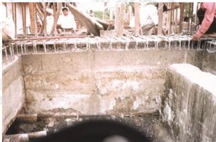
Casting of 1200mm x 900mm Beams
