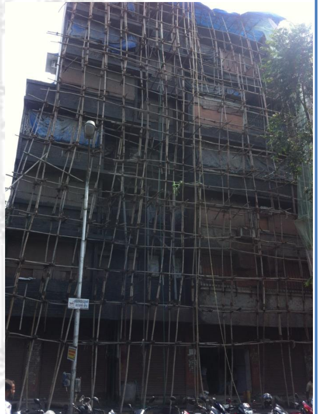
Completion of 1 st Coat Plaster North Side
