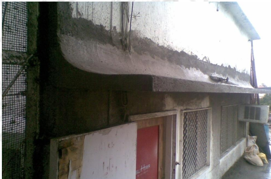
After Casting & completing of Ferrocement Chajja
