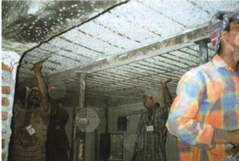
Removing Ceiling loose plaster and concrete Man chizaling
