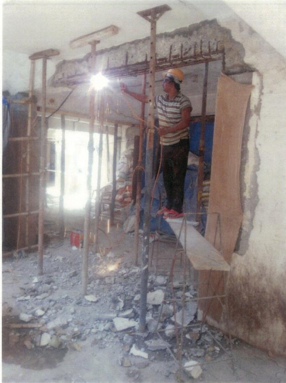
Fixing new steel bars and welding to beam
