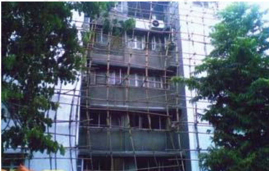
E/W Finish Plaster with White work
