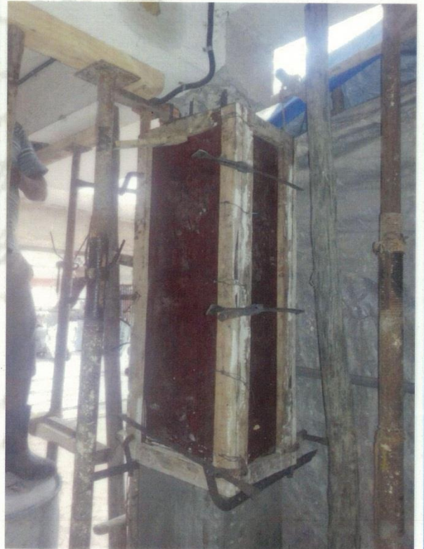
Shuttering work to colum
