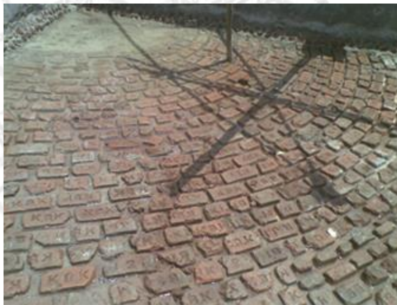
Brick Bat laid Terrace Water Proofing
