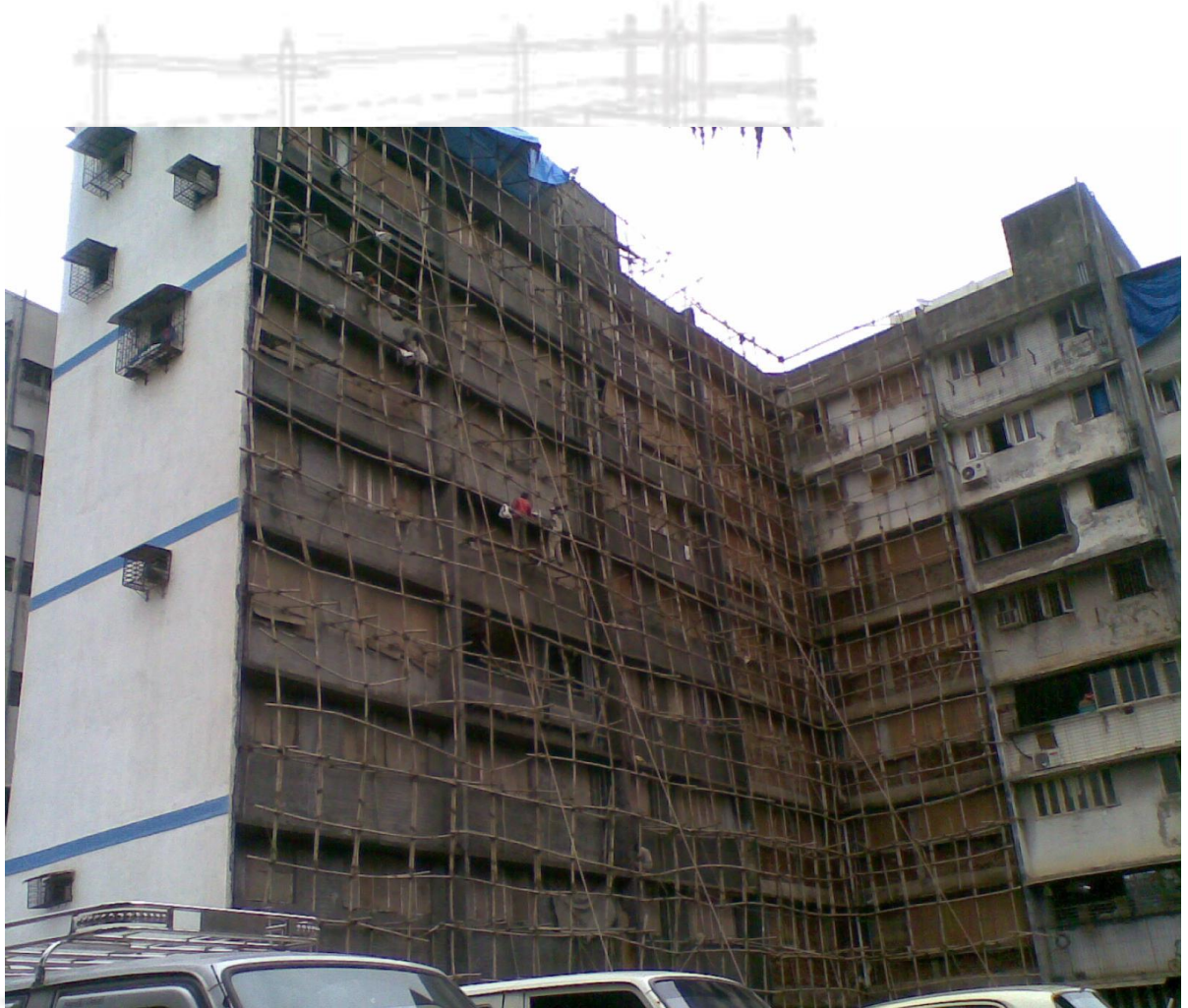
Scaffolding and Surface Preparation
