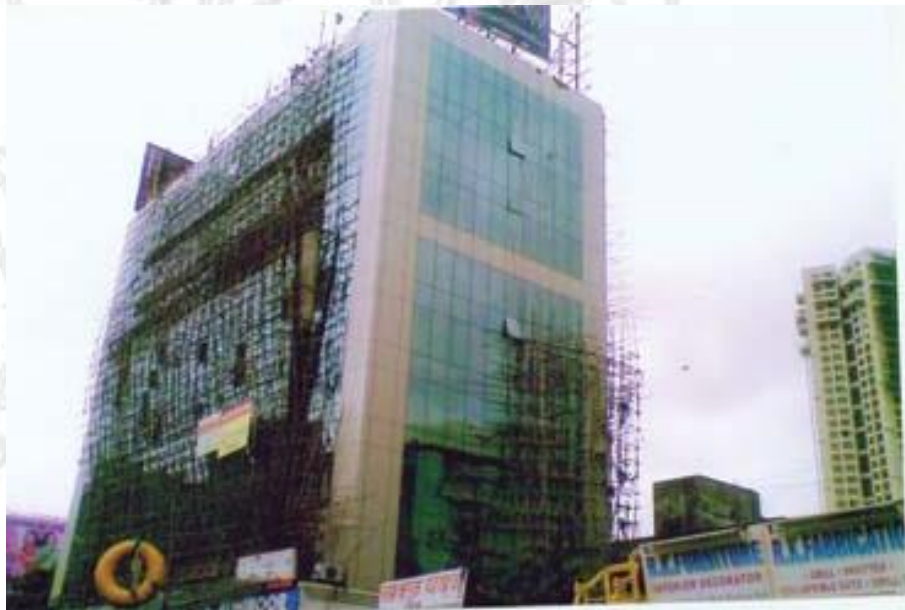
W/S Side Elevation Glazing work
