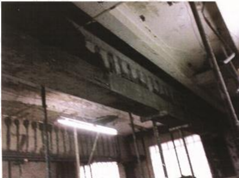
Appoxy Treatment & Centering Beam and providing Micro concrete
