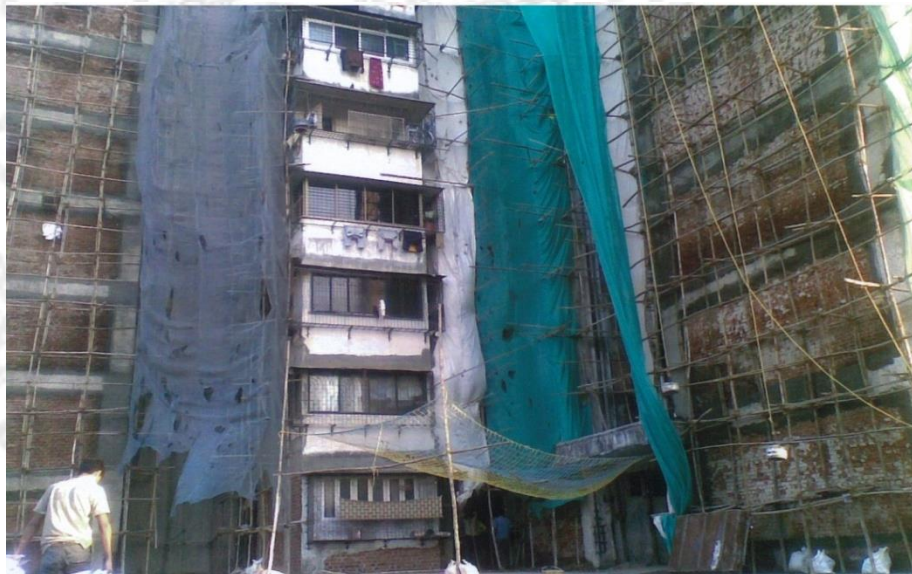
After Scaffolding and Safety measures while repairs
