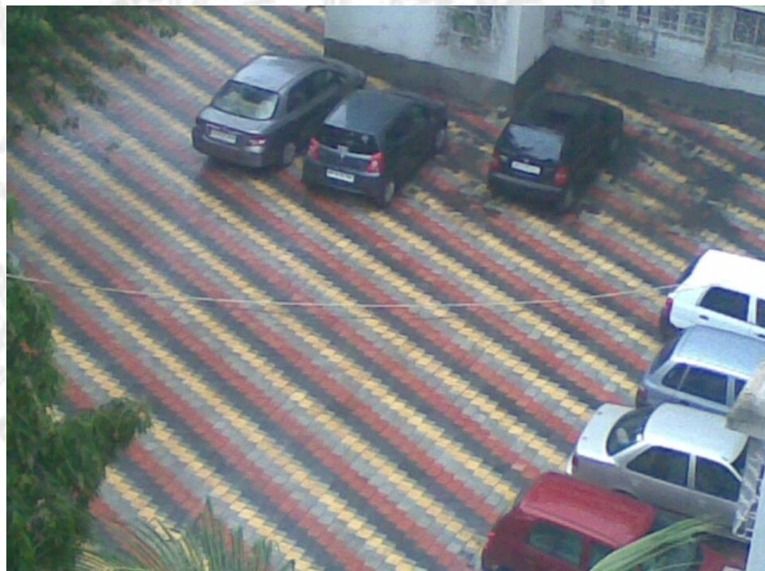
After Completion of Pavement Work
