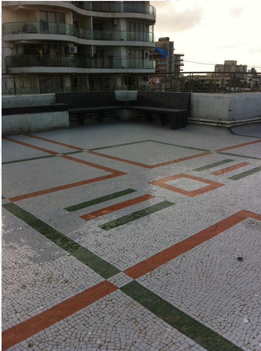
Fixing of China Mosaic Chips in Pattern
