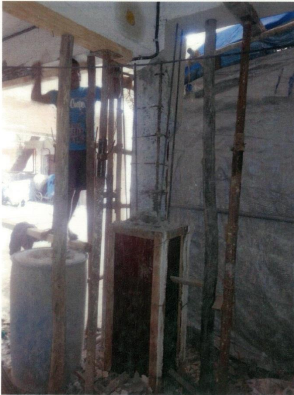
Column with Shuttering & Microconcreting
