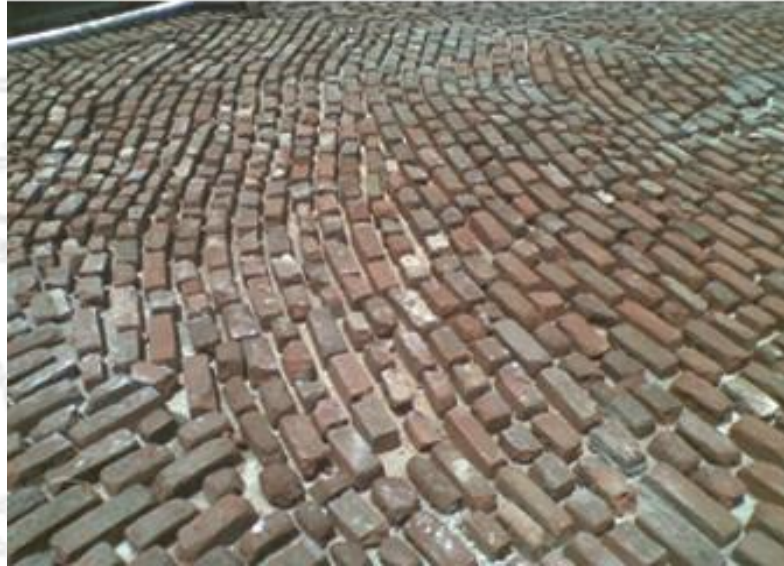
Brick Bat laid Terrace Water Proofing
