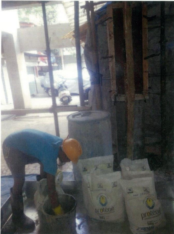
Mixing of Microconcreting
