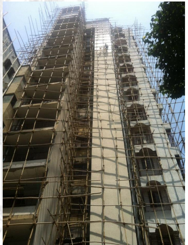
After Completion of Major Repairs and Painting
