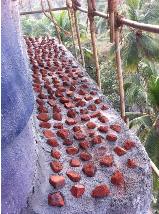
Chajja Top Waterproofing
