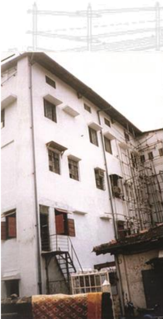
W. N. Elevation After repairs with PVC Rain water line
