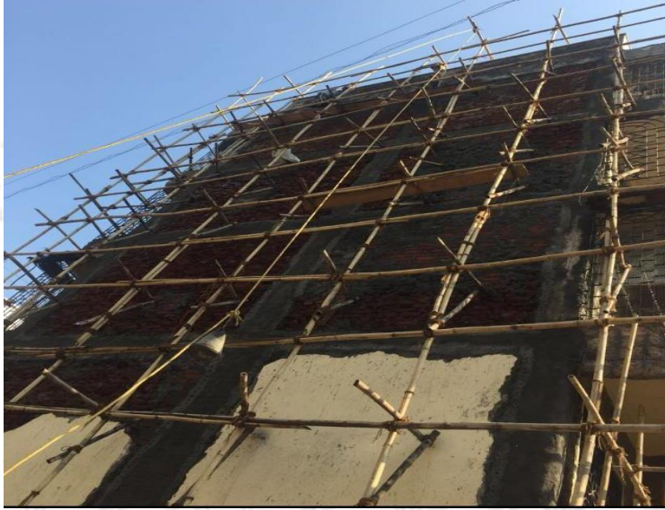
Polymer and Separation Gap Filling
