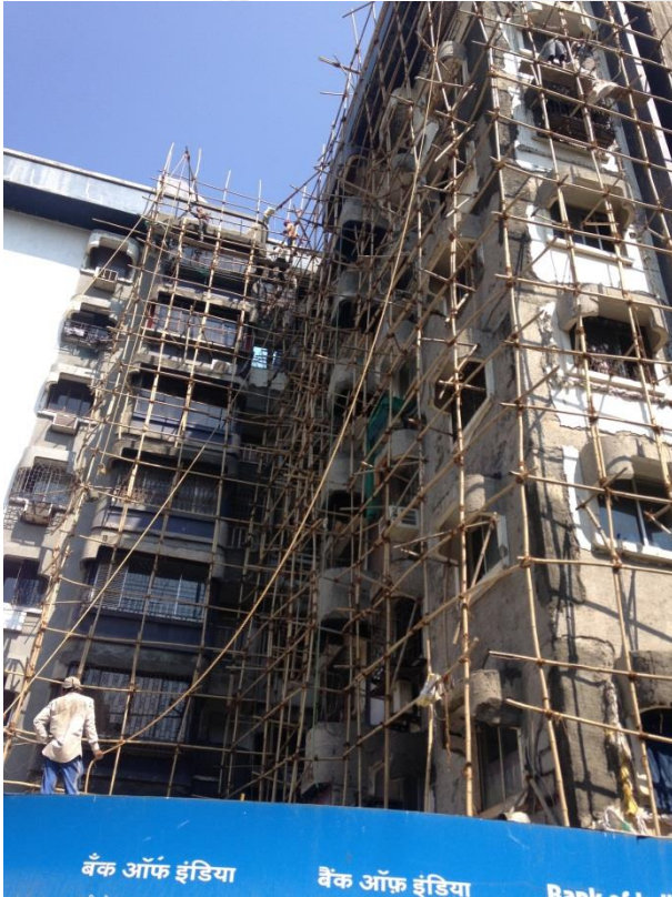
Plastering of Chajjas & Wall
