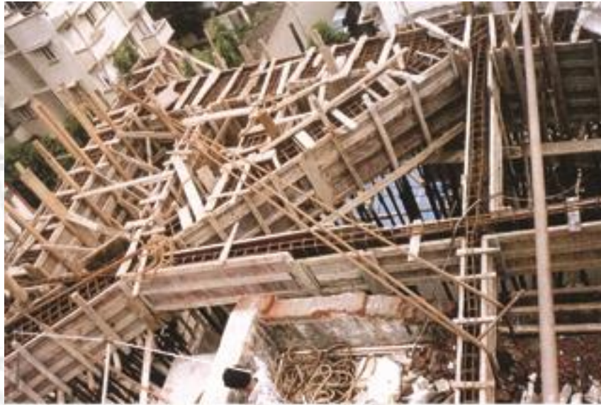
Casting of 1200mm x 900mm Beams
