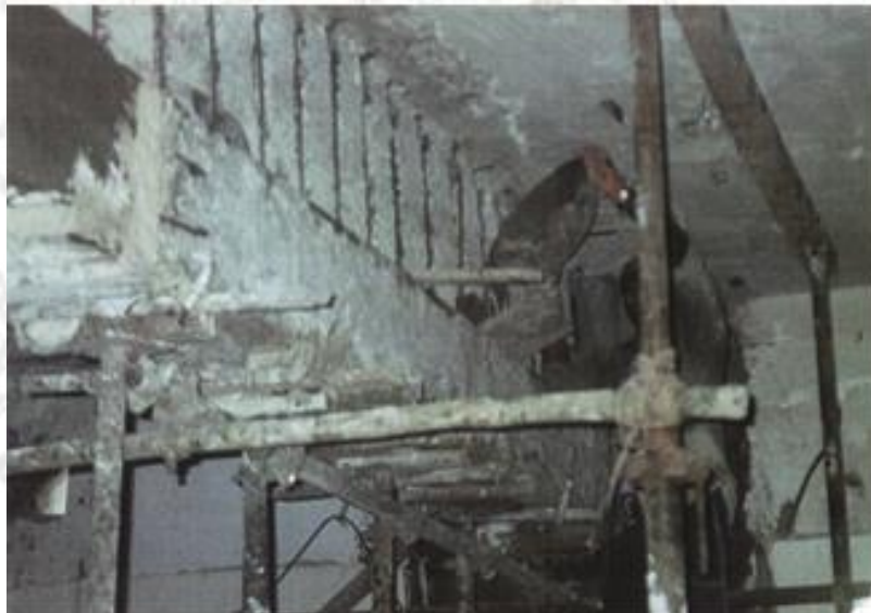
RCC Beam Centering both side applying P.M.M.
