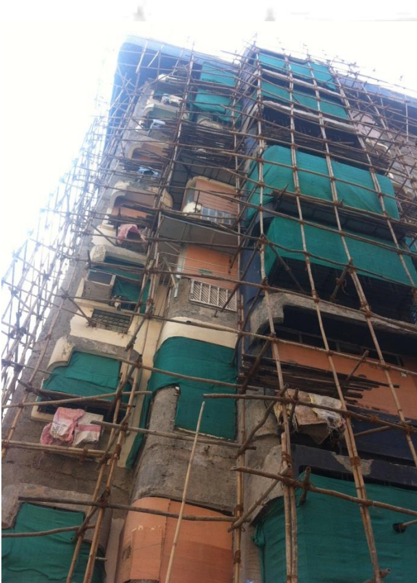
Making of Bamboos Platform
