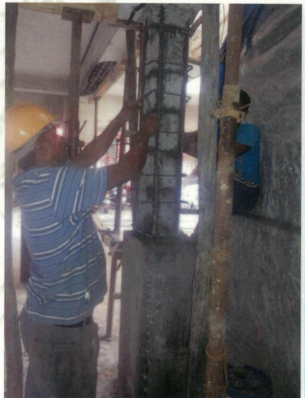
Steel Bending & Tying in position
