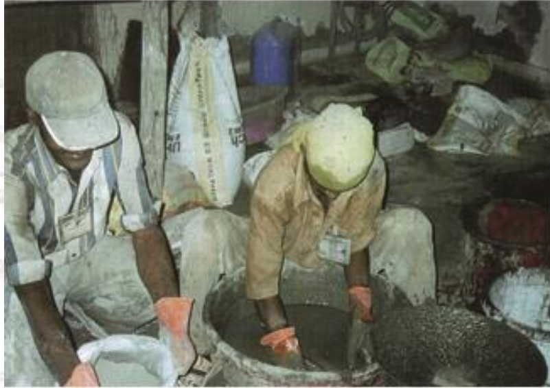
Mixing Polymer Mortar
