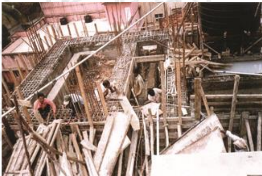
Casting of Tie Beams of Service Slab Size 1200m x 900m
