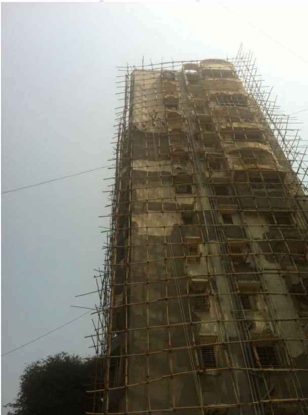
Final Finishing Plaster
