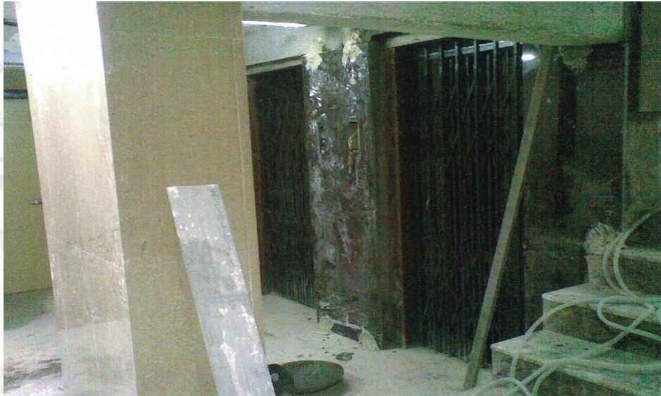
Interior Work (Cladding of Granite of the Lift Entrance)
