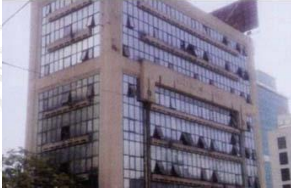
N/W Side Before repair and Glazing work
