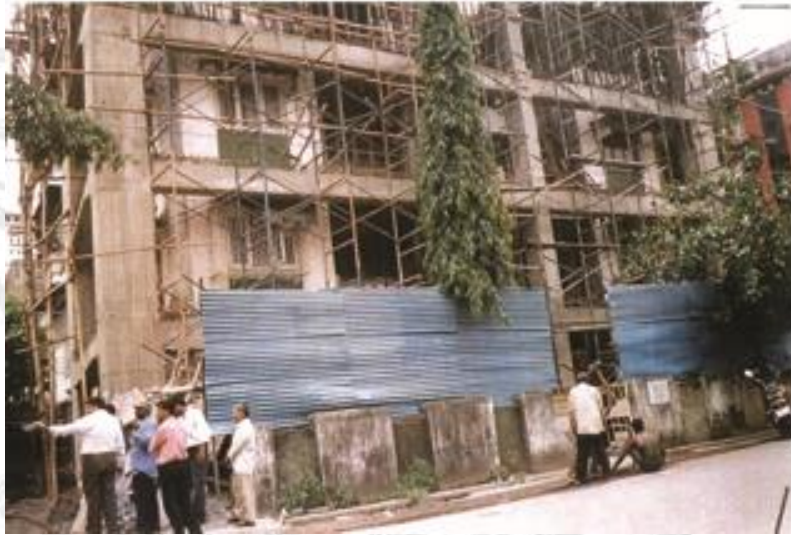
External Columns & Beams
