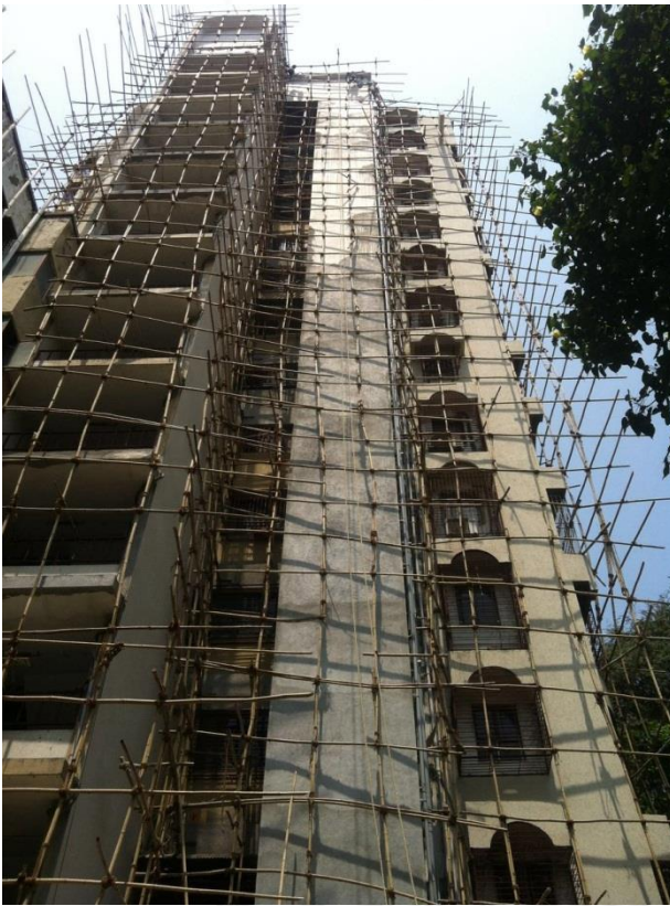
Final Finishing Plaster
