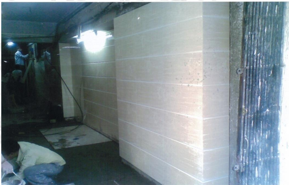
Interior Work (Fixing of wall & Floor Tiles of Front Lobby)
