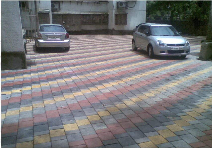
After Completion of Pavement Work
