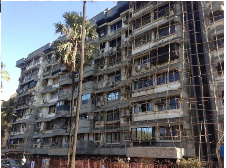
Opening of Scaffolding
