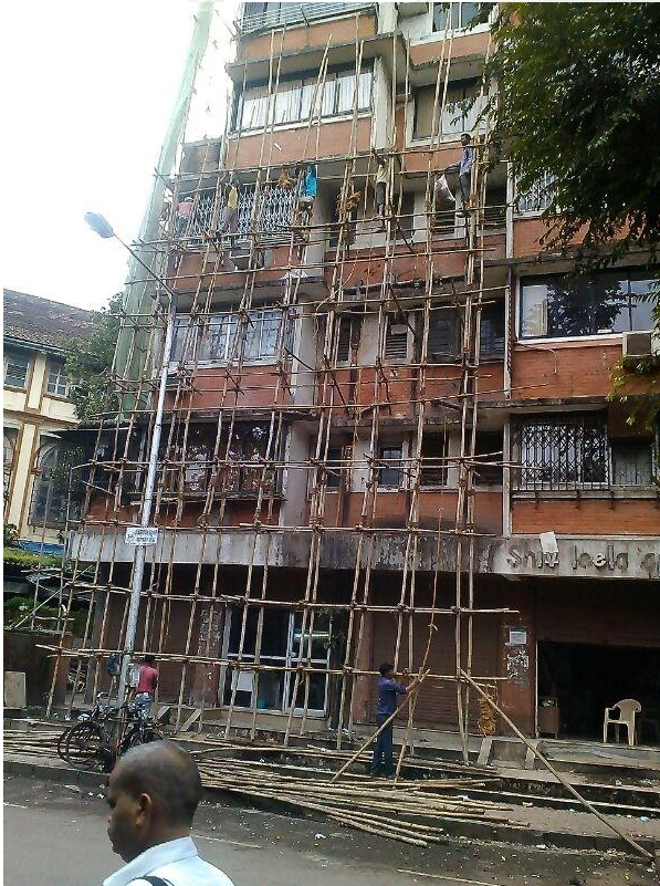
Erecting Scaffolding North Side
