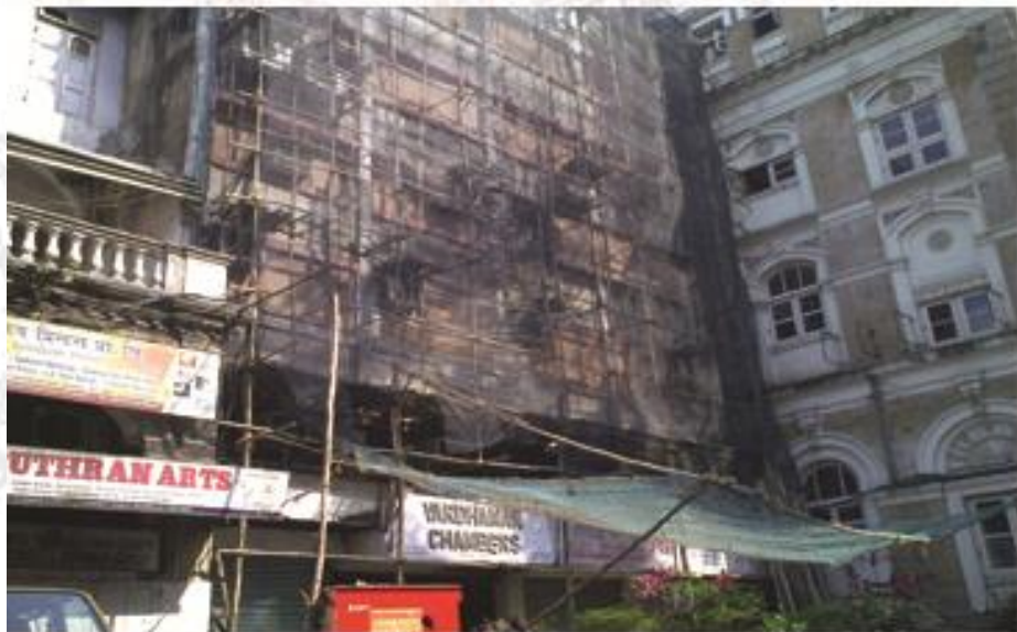
After Scaffolding and safety measurement while repairs
