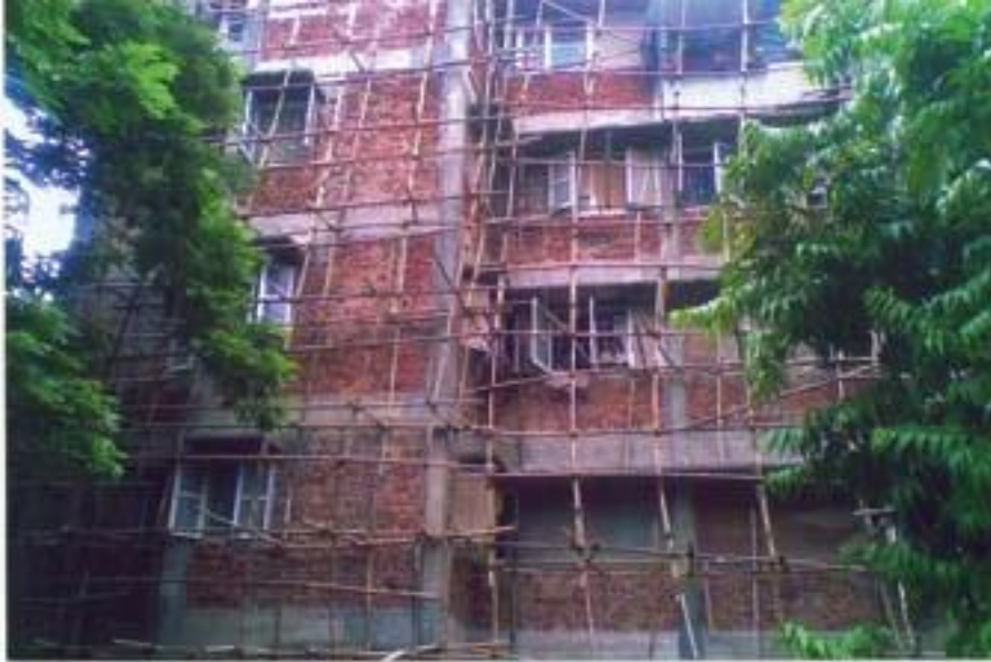
E/N Side Structural Repair Work
