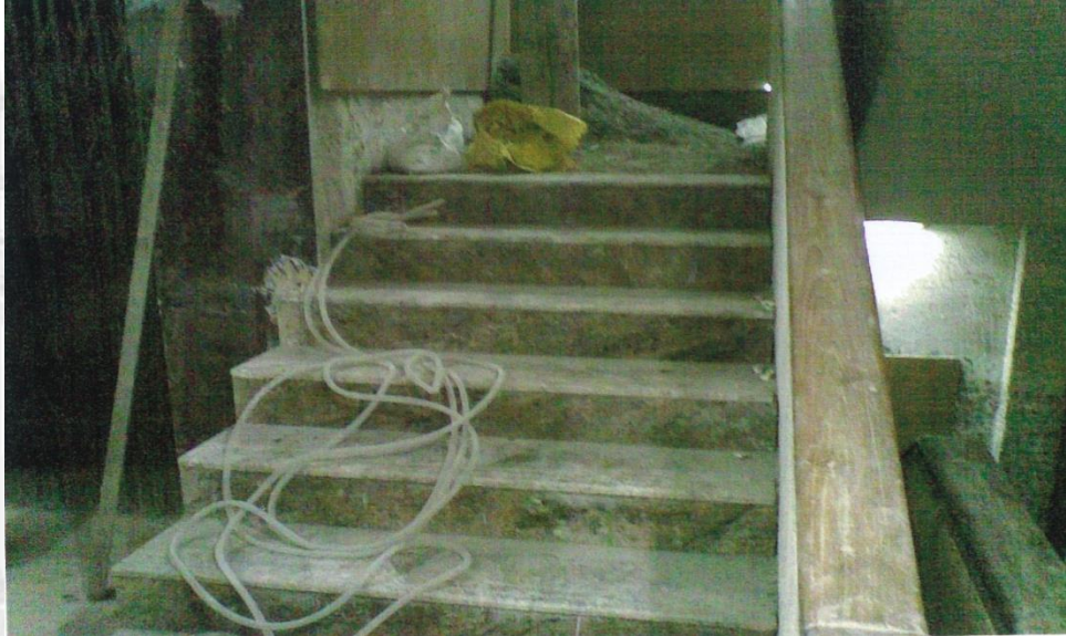
Interior Work (Fixing of Raster & Tappa)
