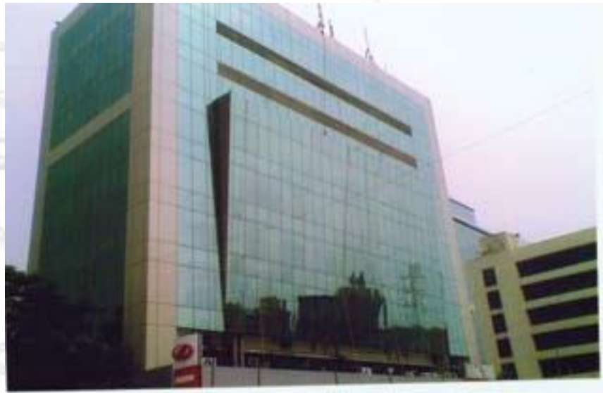
N/W Side Elevation of Glazing work
