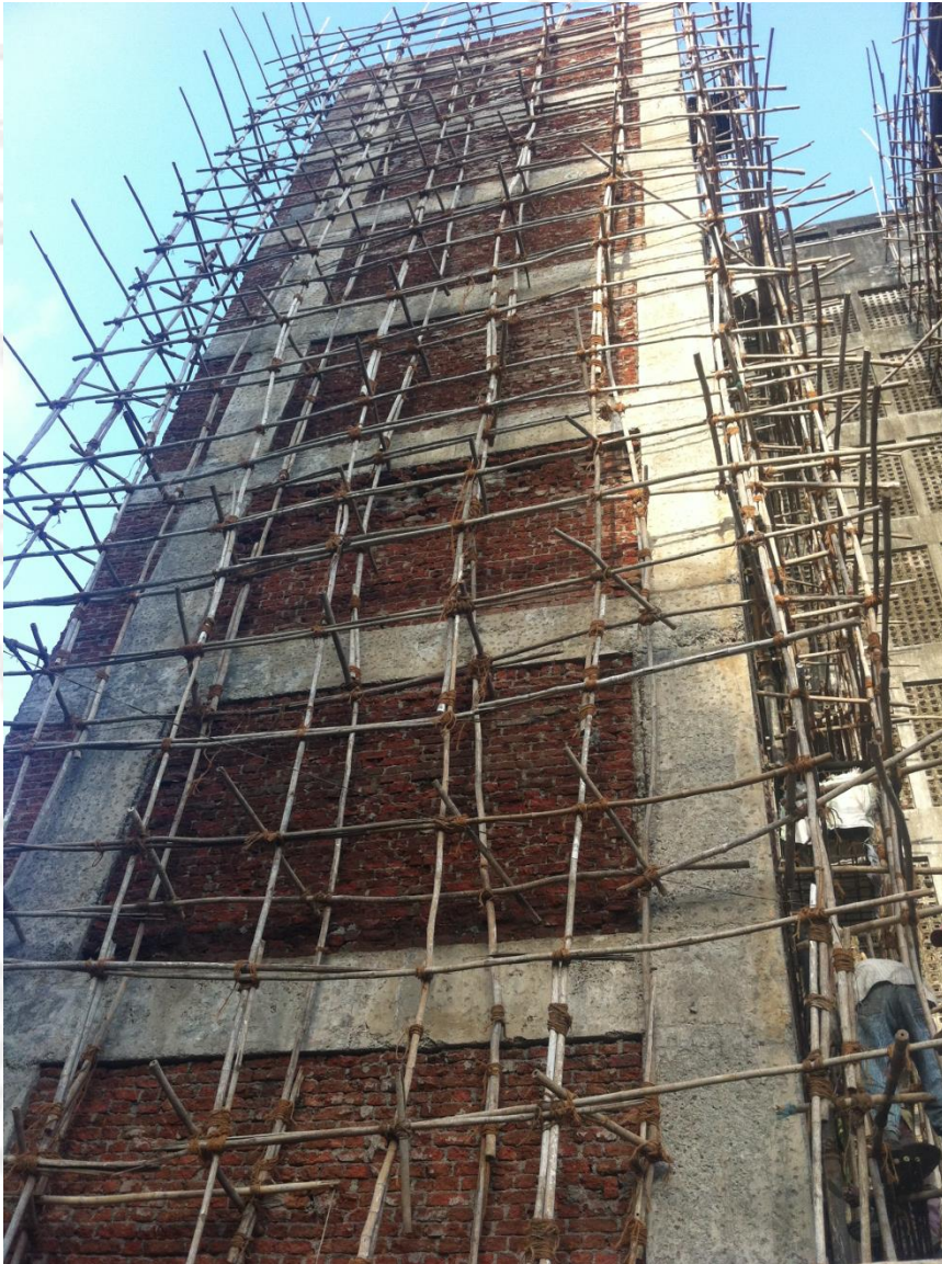
Breaking of External Plaster
