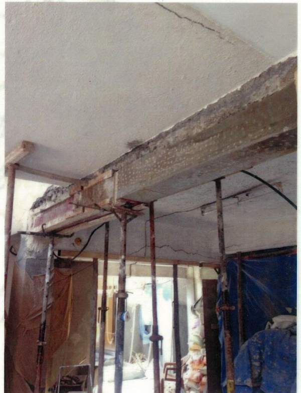
Shuttering & Microconcreting to Beam
