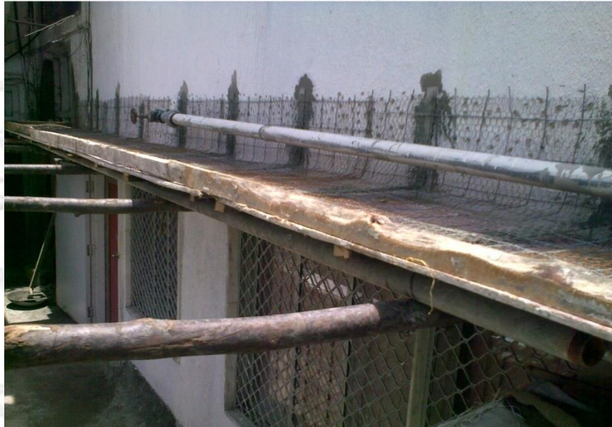
Shuttering work being done for Ferrocement Chajja
